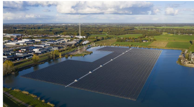
Floating solar Source: BayWa
